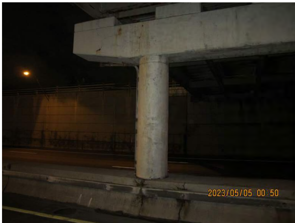
PHOTO 7: LOCATION: PIER DESCRIPTION: GENERAL CONDITION PHOTO
