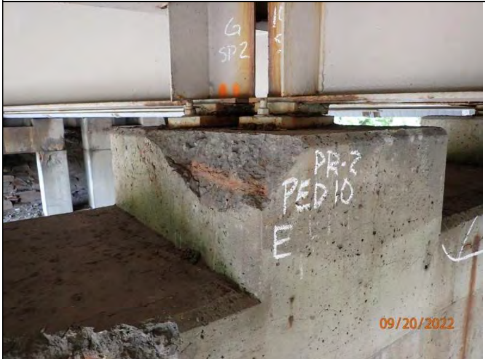
Photo Number: 40 Photo Filename: 40-Right face of G-10 Pedestal at PR-2 spalled
