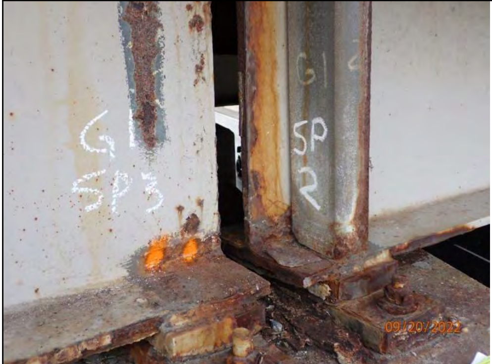
Photo Number: 10 Photo Filename: 10-Tube repair and active corrosion in lower
