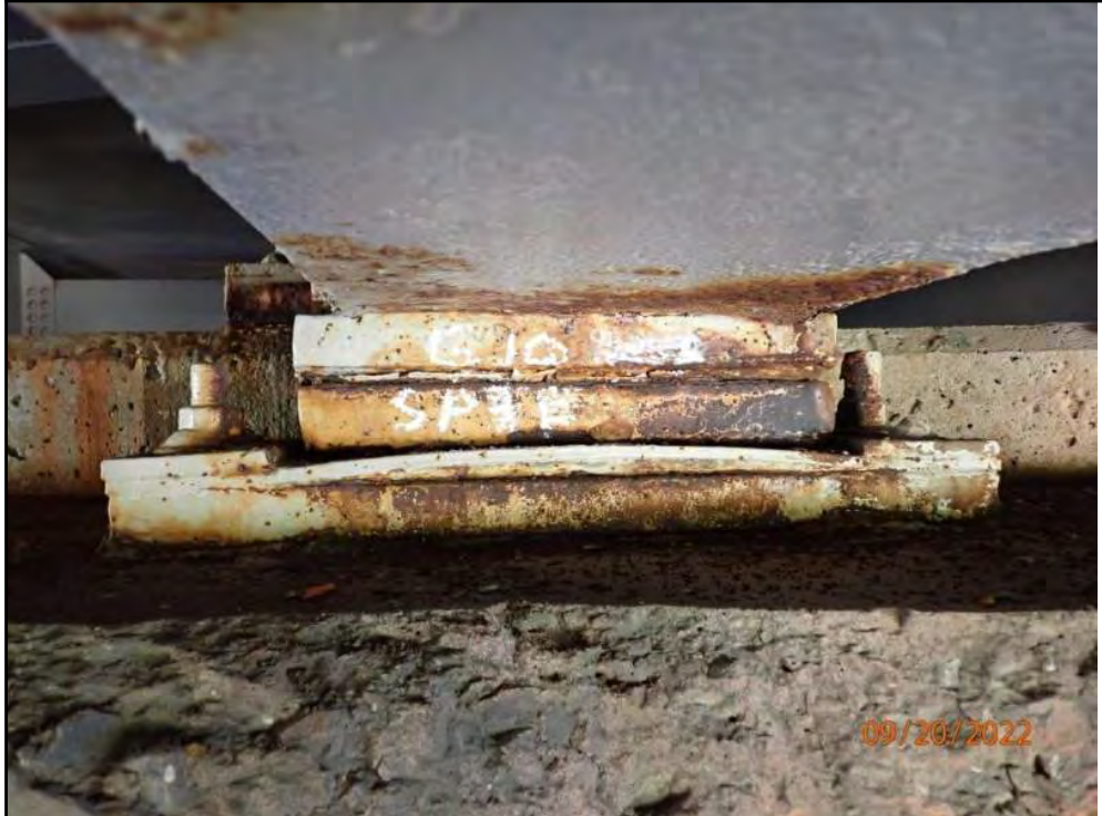
Photo Number: 28 Photo Filename: 28-Typical condition of sliding Bearings at
