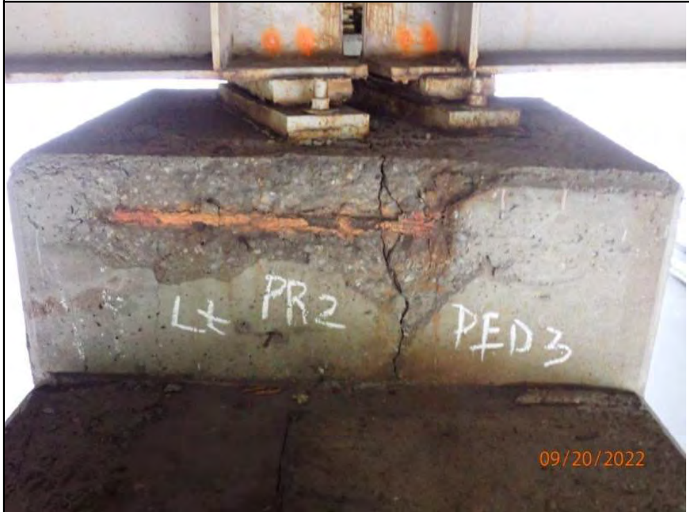
Photo Number: 39 Photo Filename: 39-Left face of G-3 Pedestal at PR-2 spalled
