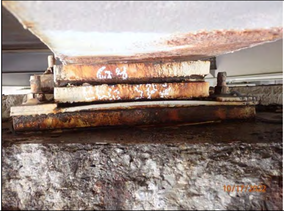
Photo Number: 27 Photo Filename: 27-Typical condition of sliding Bearings at
